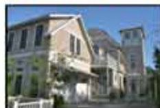
19 S. Watch Tower Lane 5 Bedrooms • 5.5 Baths 4,029 SQ FT • $2,195,000 Over 1000 SF of outside docking.
